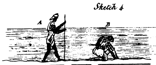
Method of extracting the Kankar near the centre of the river
